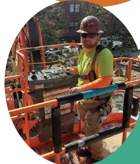
Dylan McHargue Portland Carpenters
